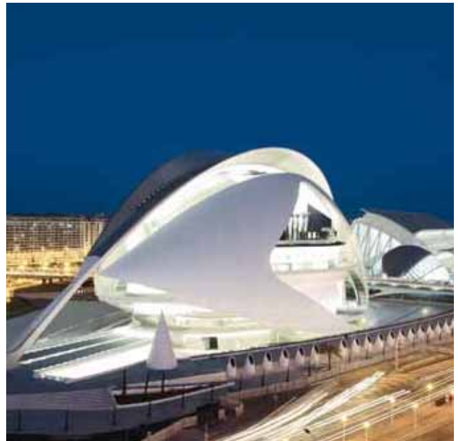
The Palau de Les Arts in Valencia – one of the largest opera houses in the world. The lighting director opted for OSRAM QTi DALI control gear for its outstanding performance.
